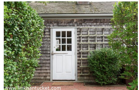
Back door on Shell Street with small brick patio and access to crawl space.
