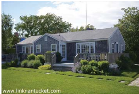
Exterior Showing Side B
