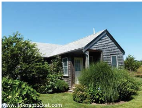
Porch off BR (2) Cottage
