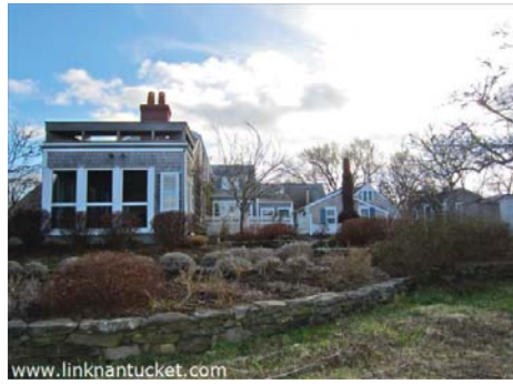
Rear of house
