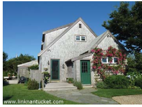
East side with access to the Kitchen & basement
